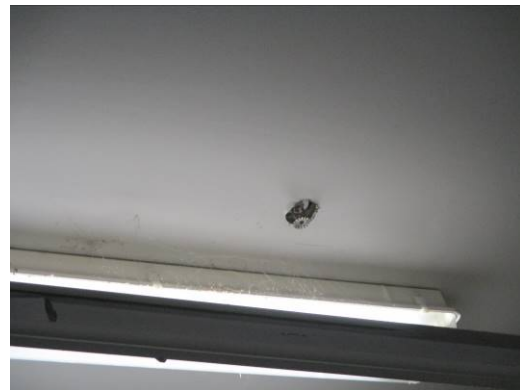
Pendent sprinklers missing escutcheons
