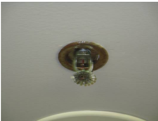
Typical semi-recessed pendent sprinkler
