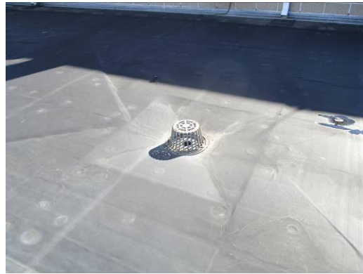
Typical roof drain
