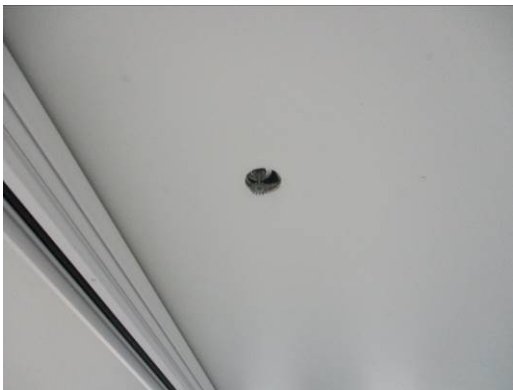
Pendent sprinklers missing escutcheons
