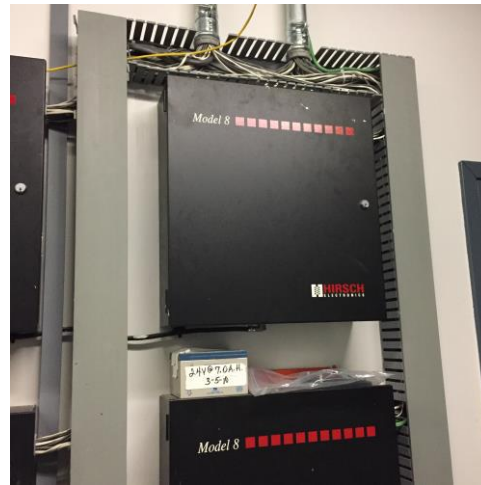
Hirsch System Being Replaced
