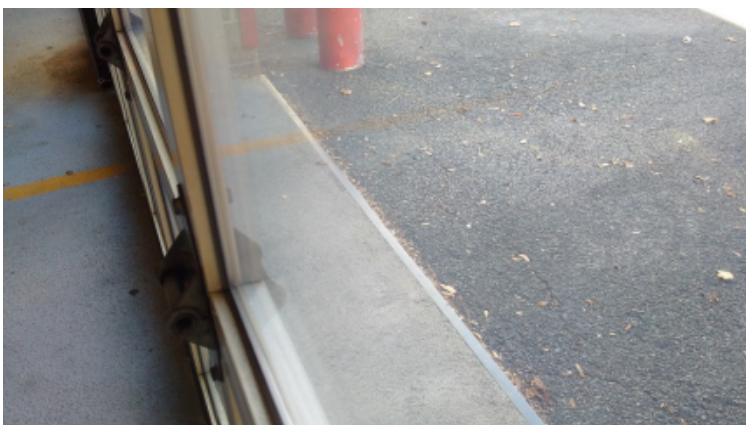
Photo 4, Grade Difference at Threshold
